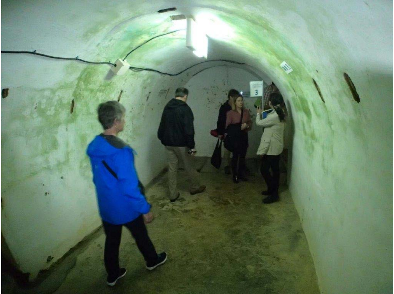
The staff room where Rear Admiral Ota pulled the pin on a grenade. You can see shrapnel splatters on the rear walls.
