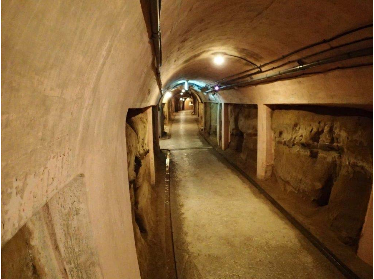
A highlight was a tour of the Navy underground headquarters, cut into sandstone.
