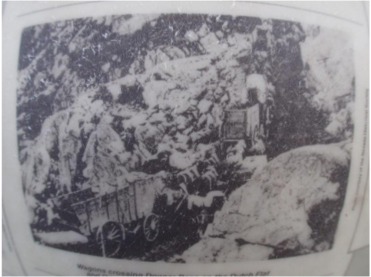
The pass, being solid granite and very steep, was a very tough nut to crack. I've been wanting to visit this site for decades, since I read a book about it.
