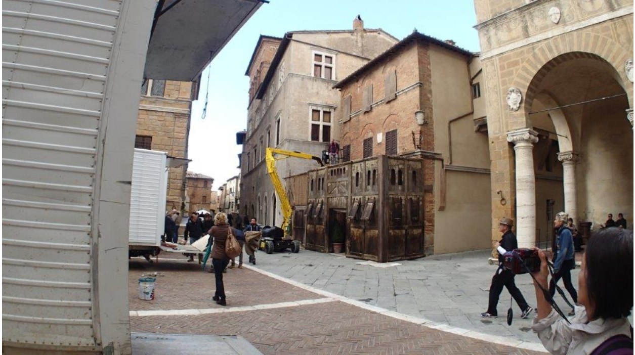
The central square was being made over for a TV series on the Medicis, who bankrolled the Renaissance. Dustin Hoffman is in the cast. The wooden extension was being constructed.
