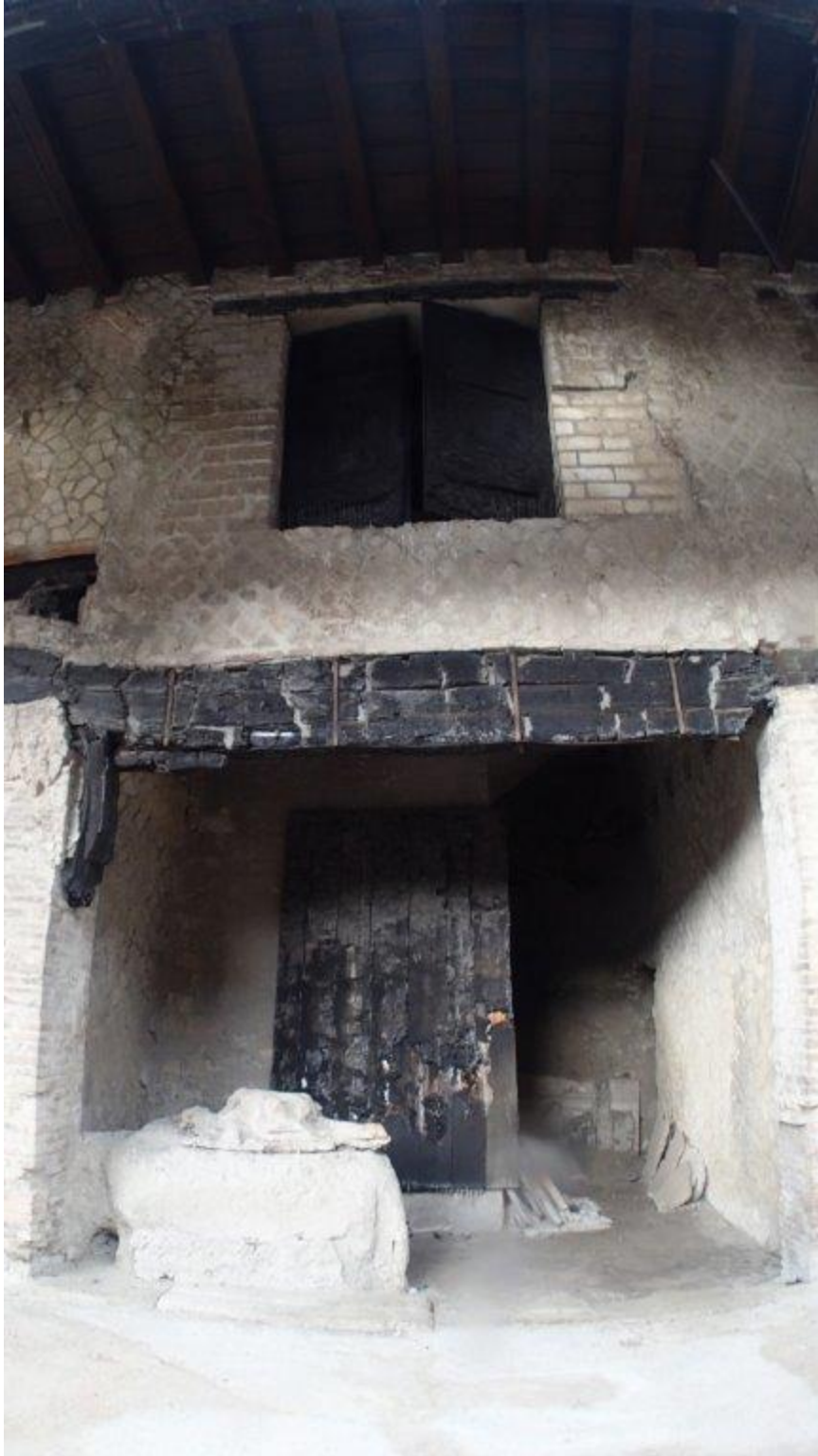
Also carbon remained. The milling in the boards on the door was just as straight and true as today.
