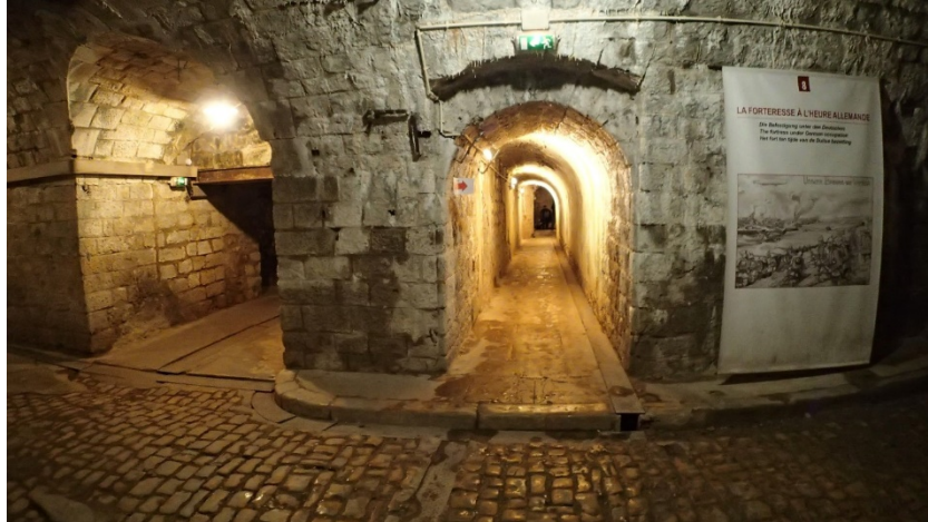
Amazingly, the underground tunnels and living quarters etc were still intact.
