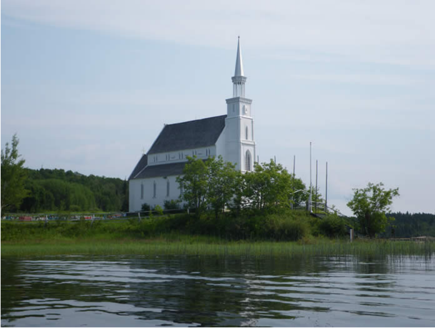
Just a mile down is the oldest structure in Saskatchewan, Holy Trinity Church built between 1854-60. It's kept in excellent condition.
